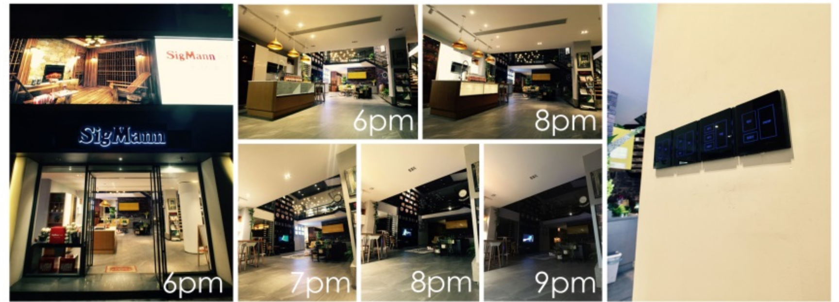
light mode being automatically changed by timer control panels
